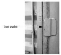
Using both hands, secure the device on the left door until it is flush.
